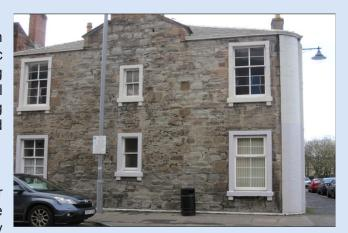
The character of this building has been adversely affected by the replacement window on the bottom right which uses uPVC, sandwiched astragals and a visible trickle vent.
