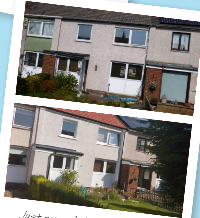
Just some of the Housing Quality and Maintenance work carried out throughout the year
