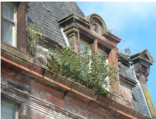
Photo 1: Dormer at east corner of south section
