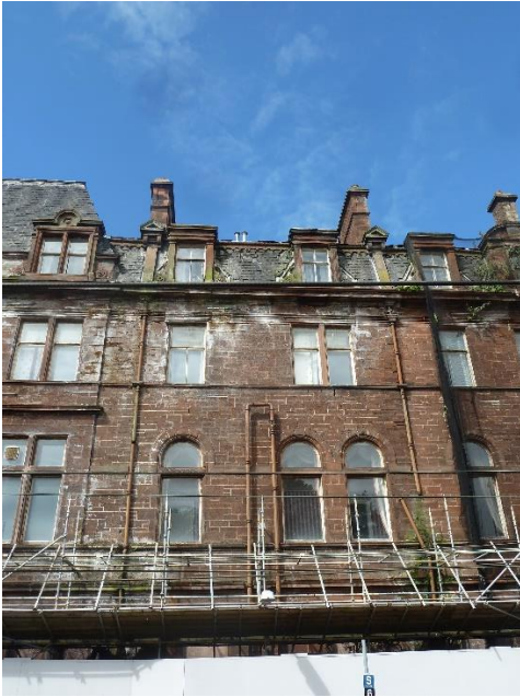
Photo 4: Efflorescence – East Elevation
