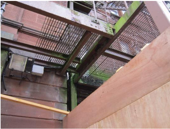
Photo 7: Escape Stair – west elevation
