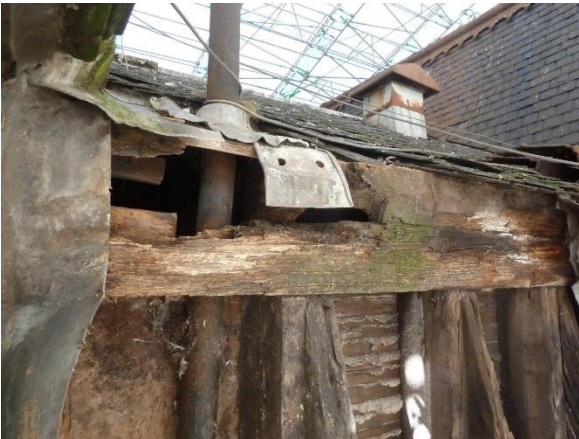
Photo 2: Roof Eaves Beam – East Elevation
