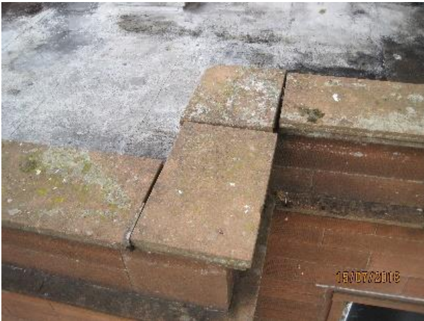
Photo 6: Loose Capping Stone – south/west corner
