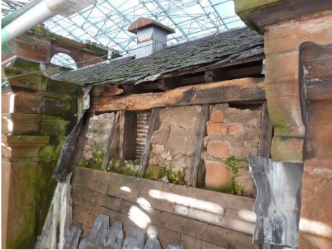
Photo 5: Lower mansard – east elevation
