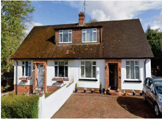
1.5 STOREY SEMI-DETACHED HOUSES
