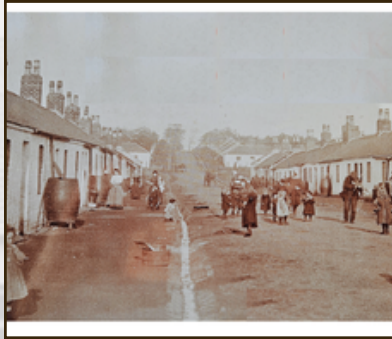
THE VILLAGE IN 1930 WITH THE NEW HOUSES UNDER CONSTRUCTION IN THE BACKGROUND
