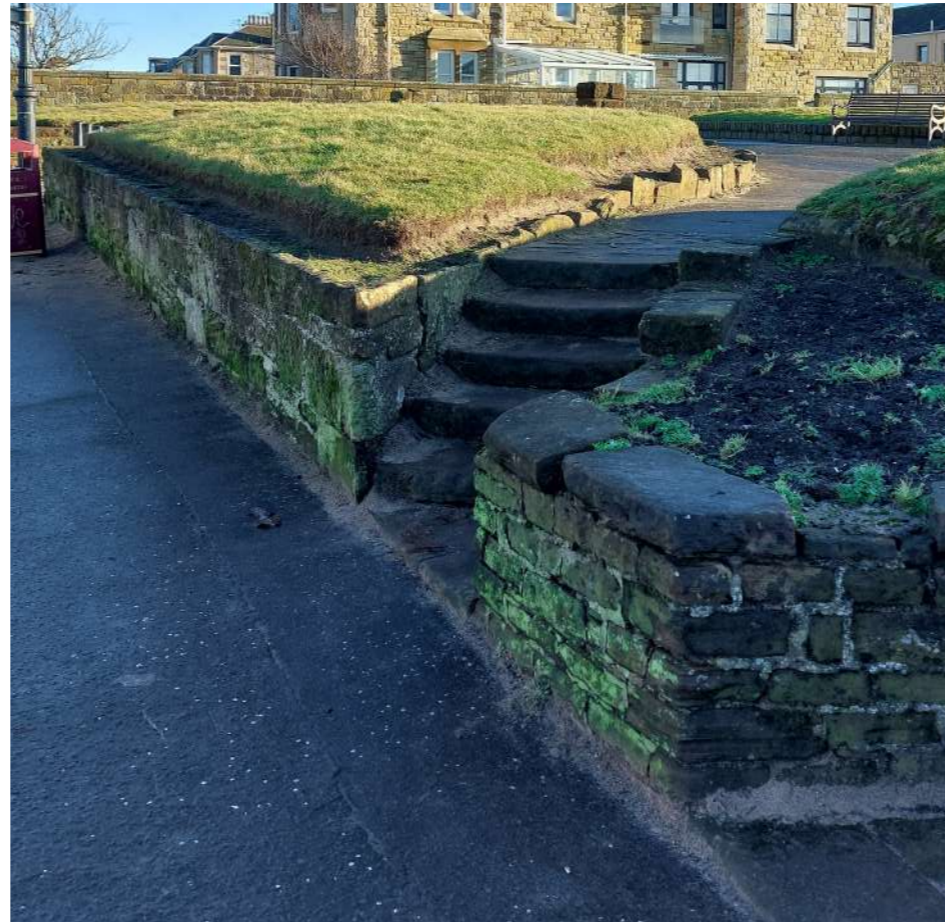
Poor quality accessibility
