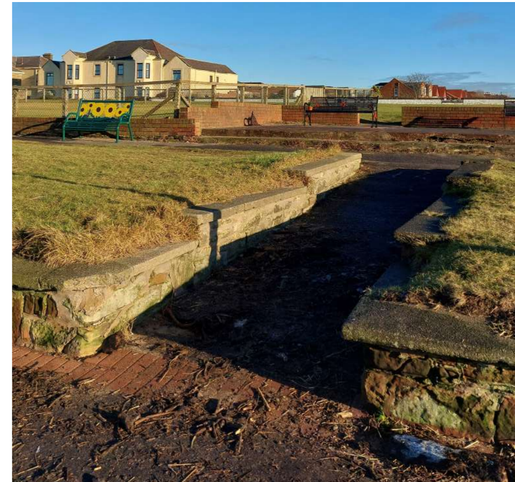
Difficult to maintain materials and details
