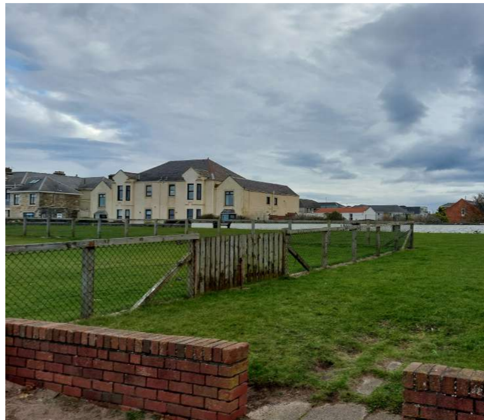
Mix of materials and poor accessibility
