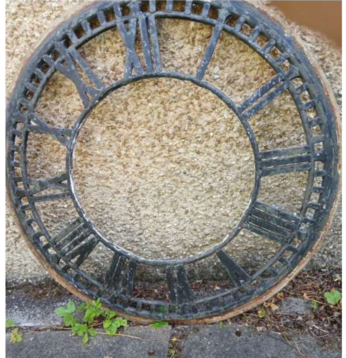
Existing clock dial, photo provided by H.E Weir & Son
