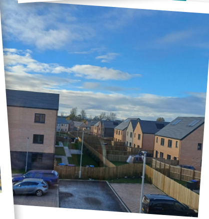
New Build Progress
