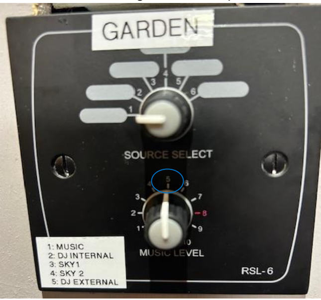
Photo 4.3(b) and (c): Garden speaker sound controller, setting '4' and '5' outputs 30/07/25
