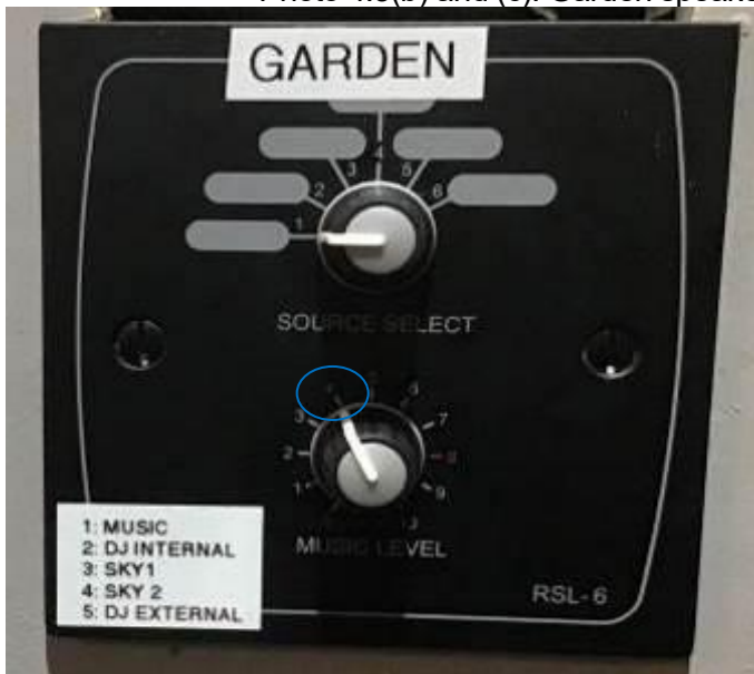
Photo 4.3(b) and (c): Garden speaker sound controller, setting '4' and '5' outputs 30/07/25
