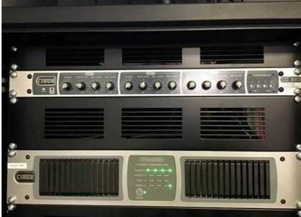
Photo 4.3(a): speaker system – Cloud CX263 mixer and CVA4250 4-channel power amp set-up 25/07/25
